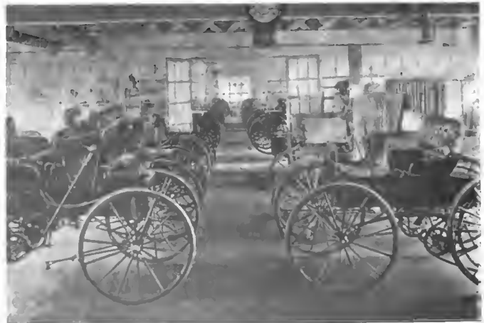
Where the Paint is Applied and the Finish Perfected.
